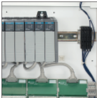
Fused outputs with terminal strip connection points
